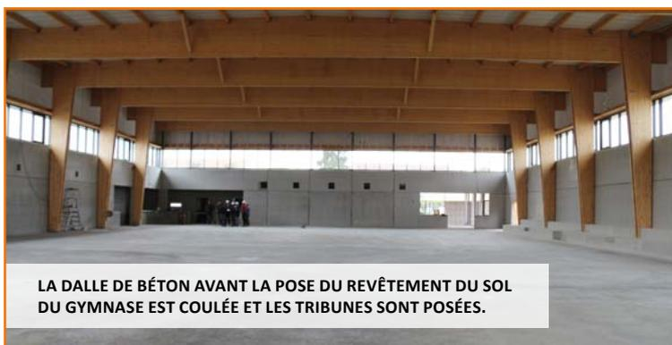
LA DALLE DE BÉTON AVANT LA POSE DU REVÊTEMENT DU SOL DU GYMNASE EST COULÉE ET LES TRIBUNES SONT POSÉES.
